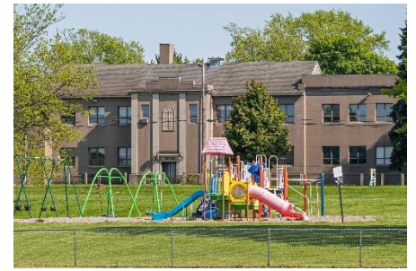
Burton School Redevelopment
