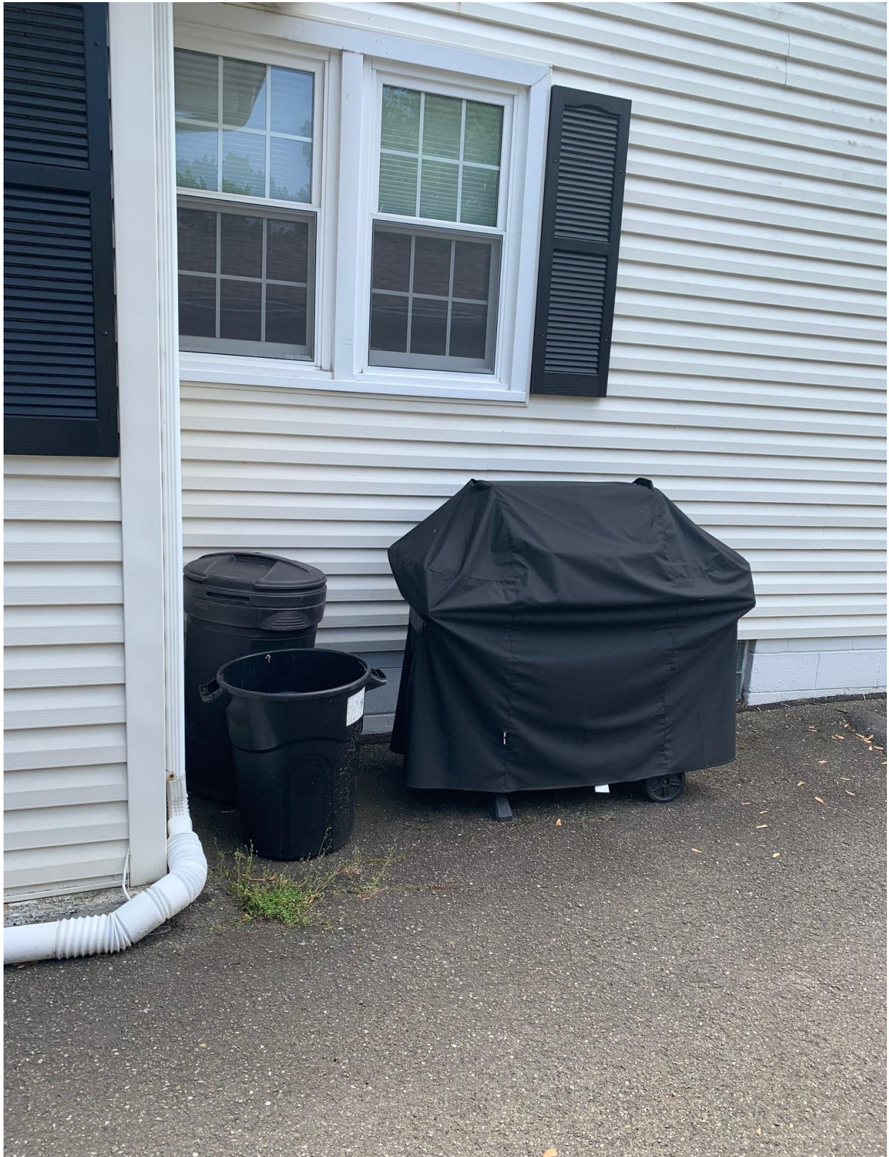
TRASH AREA- 154 ANDREWS PARK BLVD
