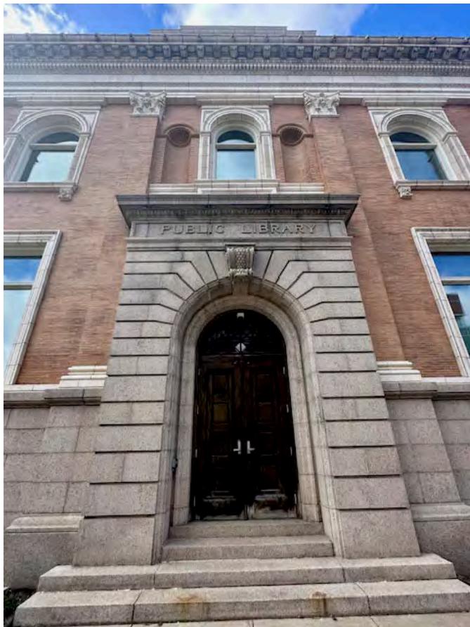
Photo. 4. Erie Main Library, Eastern Entrance. Feb., 2024. M. Falcone.
