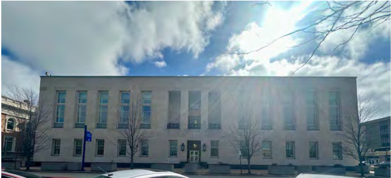
Photo. 1. U.S. Federal Courthouse, North (primary) Façade. Feb. 2024. M. Falcone.
