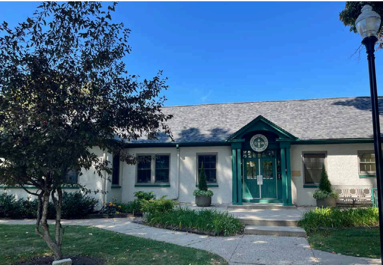
Selden Building Door faces South East
