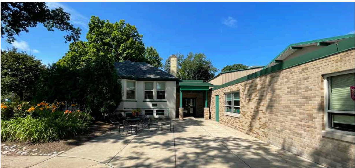
Spencer Building addition Door faces East
