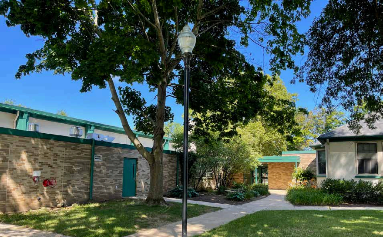
Breezeway & Back of Dining Room/Kitchen Door faces South East
