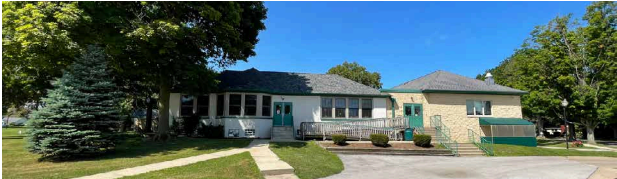
Selden Building and addition Door faces East
